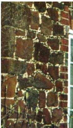
A much less usual form of construction is walls and galleting of ironstone but this can be found in the area around Borough Green near Sevenoaks. The stones are very dark brown as can be seen in the photograph on the left.
