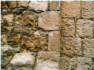
The picture on the left illustrates two forms of ragstone galleting in one building, being part random stonework of the late 18th century and part later squared and coursed work. In the centre are quoin blocks that are block bonded into the random stonework to form a corner. Galleted Kentish ragstone masonry can be found in a narrow band from Deal in the east, crossing Kent to Maidstone and Sevenoaks and heading west to Surrey.
